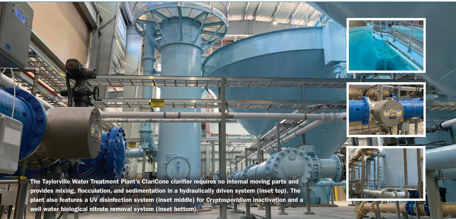
The Taylorville Water Treatment Plant's ClariCone clarifier requires no internal moving parts and provides mixing, flocculation, and sedimentation in a hydraulically driven system (inset top). The plant also features a UV disinfection system (inset middle) for *Cryptosporidium* inactivation and a well water biological nitrate removal system (inset bottom).
